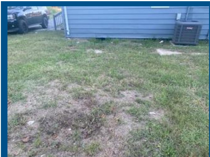
Keisha Hardy's home where the sewage is coming up into the yard. The home was purchased with no idea that the septic system was homemade and failing.
