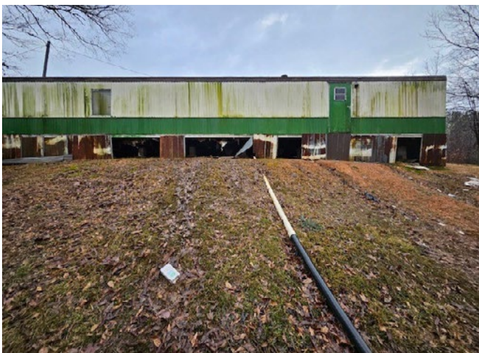
Photo 2. Examples of straight pipes and failing septic systems in the Black Belt Region of Alabama.
