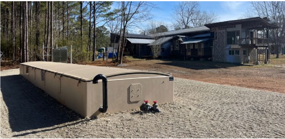
Photo 5. Modular wastewater treatment system installation at Rural Studio in Newbern, AL.
