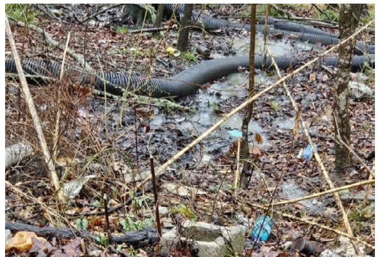
Photo 2. Examples of straight pipes and failing septic systems in the Black Belt Region of Alabama.
