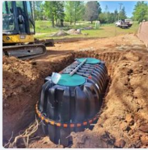
$7,500 New septic system Hickory, NC
