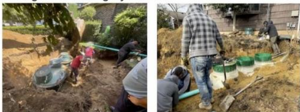
A Hydro-Action System being installed (left) and Fuji Clean (right)
