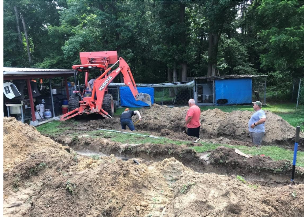
Installed new drainfield trenches
