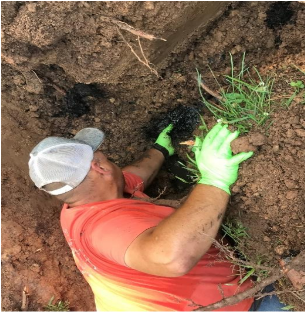
Unclogged trench & connected effluent pipe to other portion of drainfield
