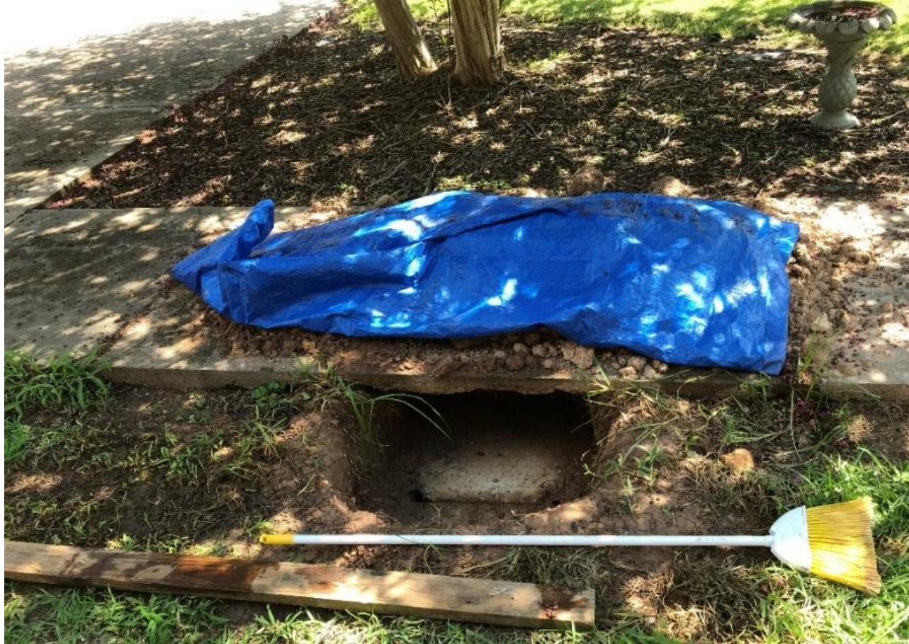
Replaced cracked septic tank lid
