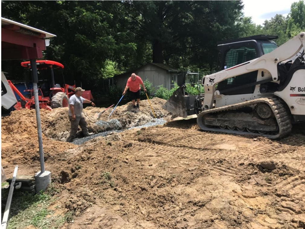
Installed new drainfield trenches
