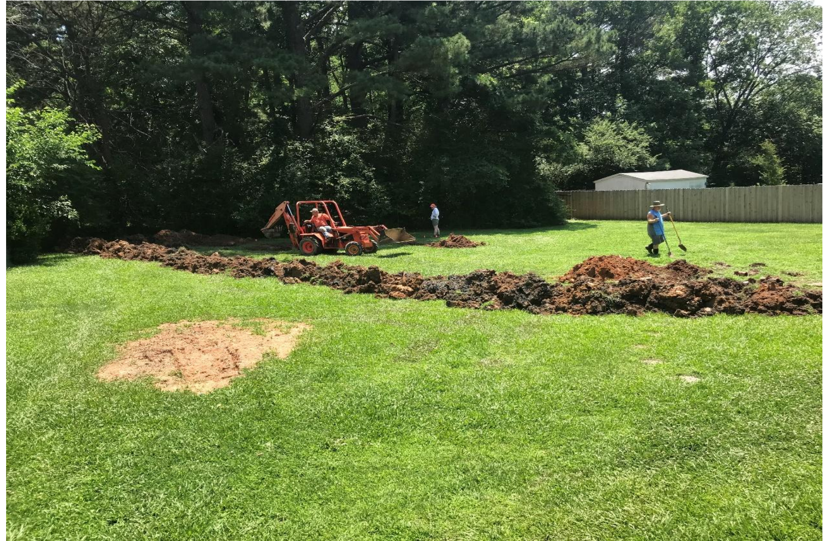
Unclogged trench & connected effluent pipe to other portion of drainfield
