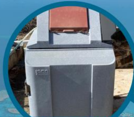
Influent Sampler: ISCO 5800 (Refrigerated)
